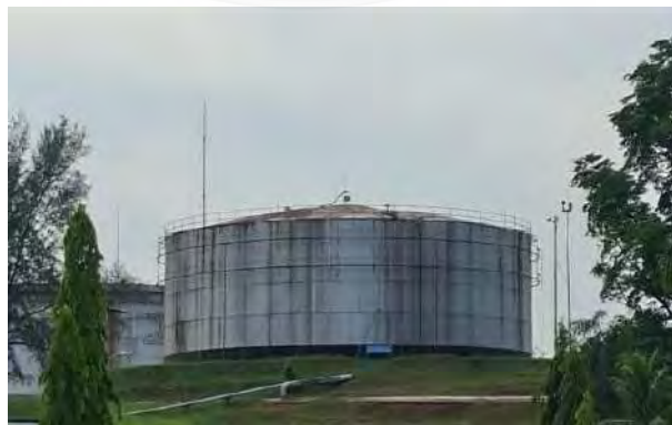
Gambar 3. 30 Main Storage Tank (Tangki Timbun Utama)
