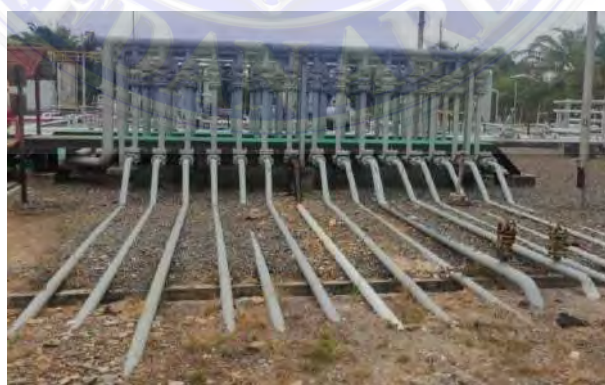
Gambar 3. 8 Manifold
