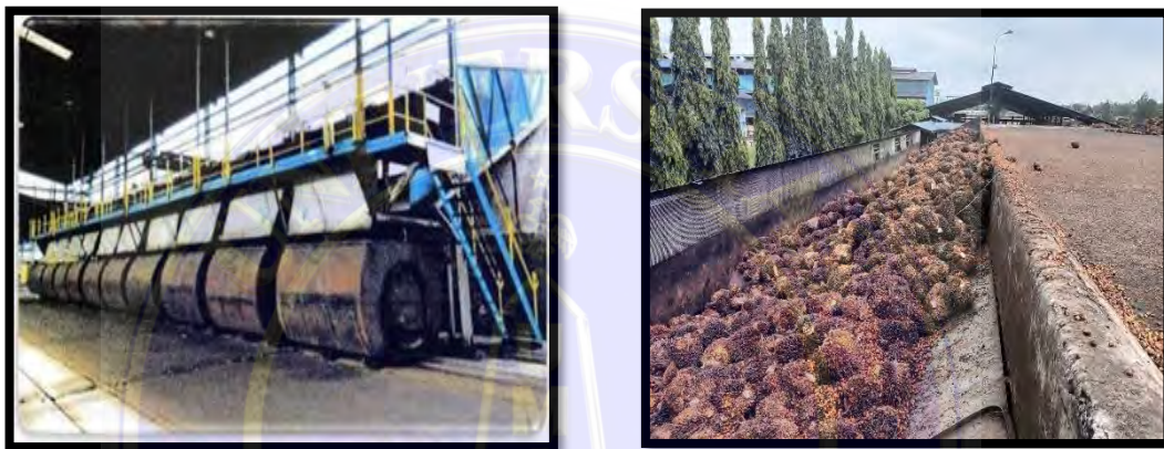
Gambar 3.3. Loading Ramp Line I Dan Line II
