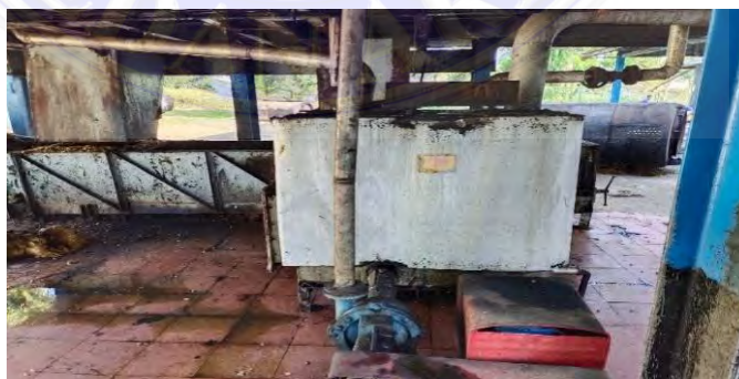
Gambar 3. 13 Crude Oil Tank 1
