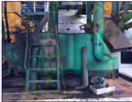
Gambar 3.2.7.8 Separating tank
