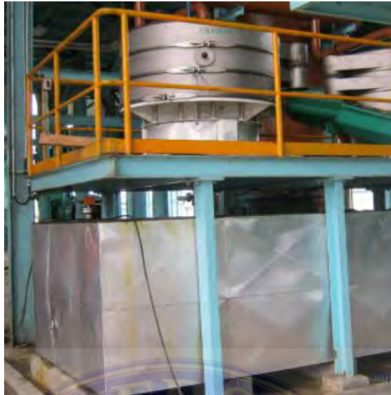
Gambar 3. 21 Crude Oil Tank
