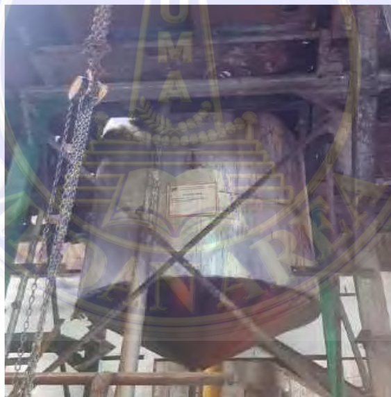
Gambar 3. 26 Sludge Tank
