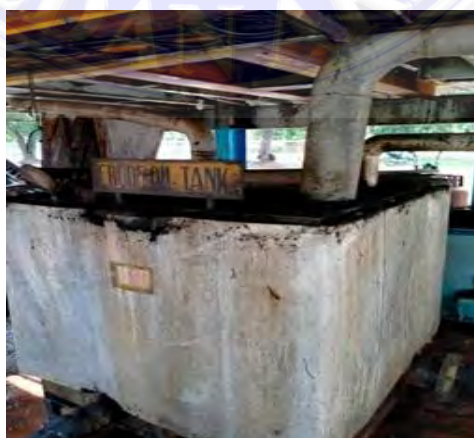
Gambar 3. 17. Crude Oil Tank
