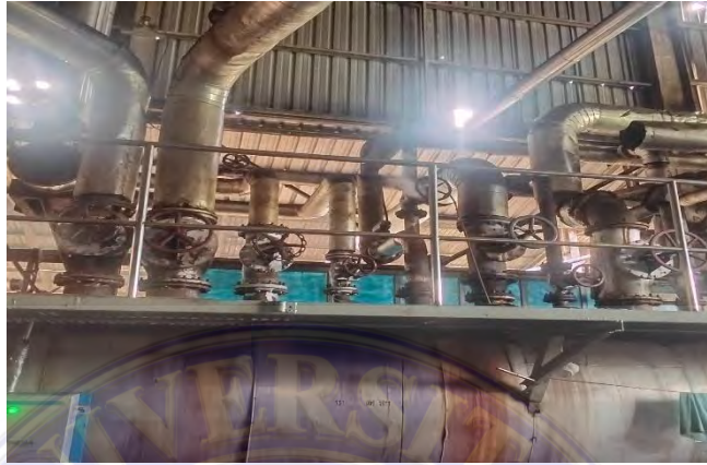
Gambar 3. 55 Back Pressure Vessel (BPV)
