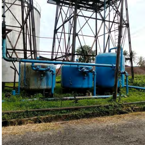
Gambar 3. 61 Sand Filter
