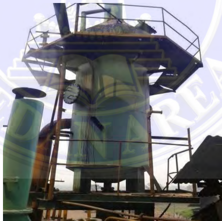
Gambar 3. 14 Flash Tank
