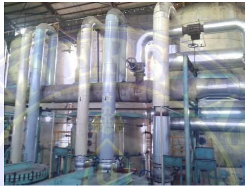
Gambar 3. 16 Evaporator
