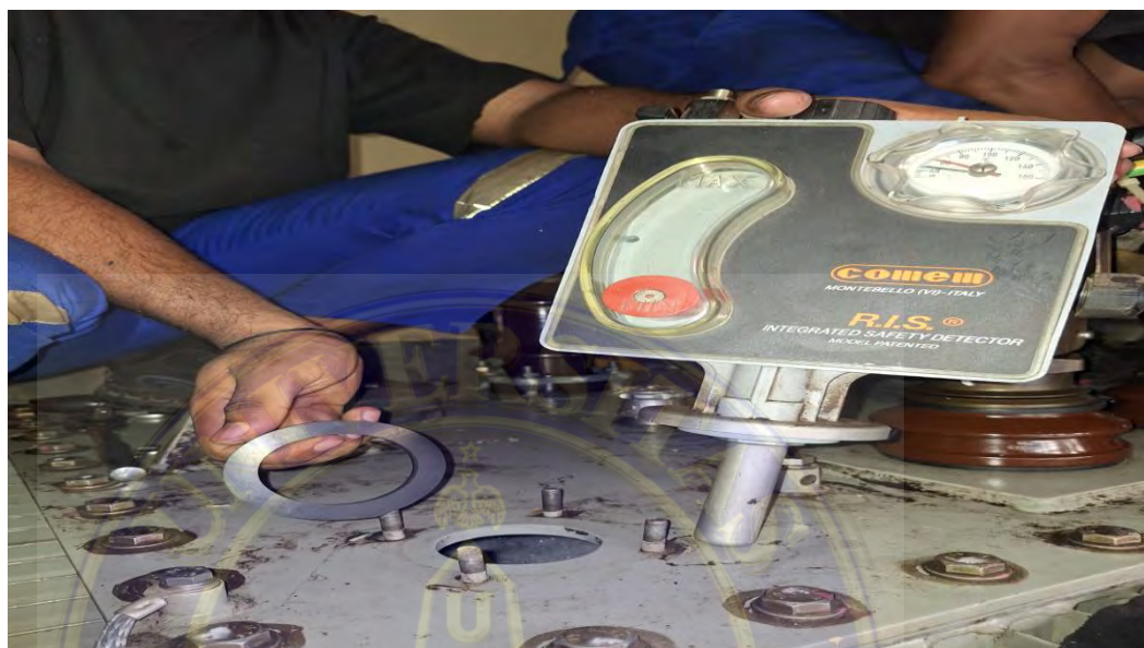
Gambar 4. 4 Pengecekan menggunakan remote integrated safety
