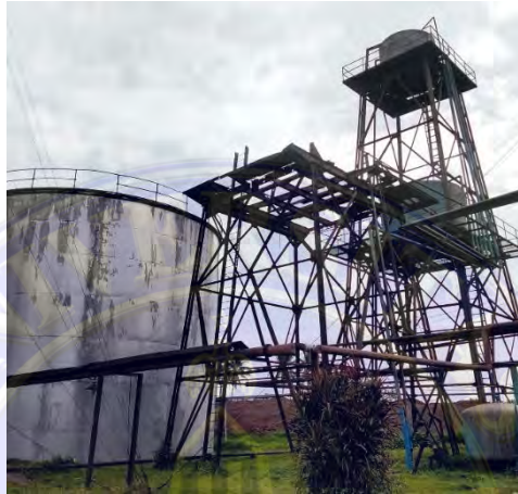
Gambar 3. 63 Water Tower Tank
