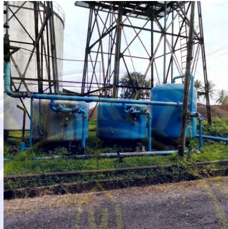
Gambar 3. 62 Sand Filter
