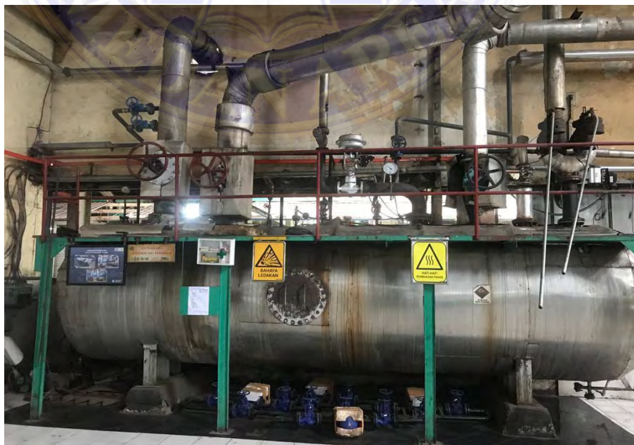
Gambar 3.58. BPV( Back Pressure Vessel )
