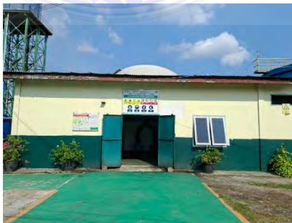
Gambar 3. 60 Water Treatment Plant
