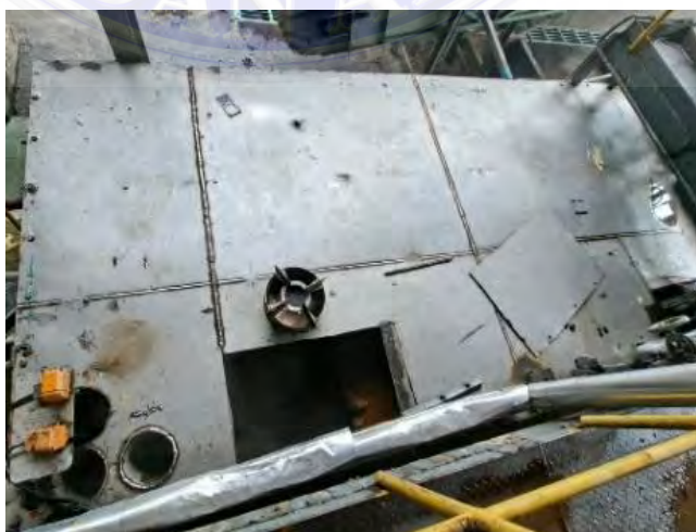
Gambar 3. 28 Crude Oil Tank
