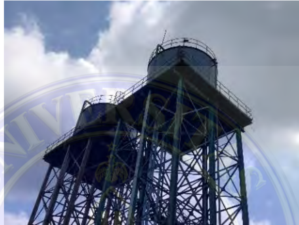
Gambar 3. 64 Tower Water Tank
