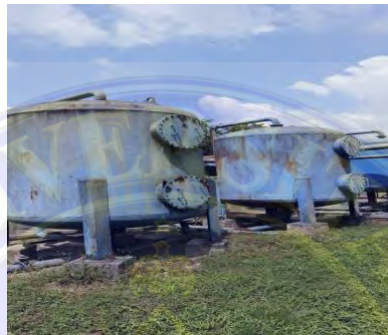
Gambar 3.54 Sand Filter
