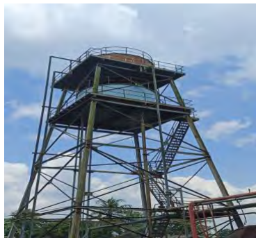
Gambar 3.55 Water Tower Tank
