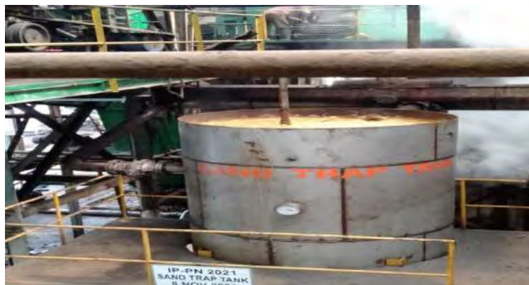
Gambar 3.13 Sand Trap Tank
