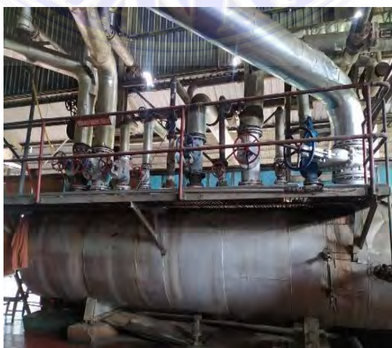
Gambar 3. 55 Back Pressure Vessel (BPV)
