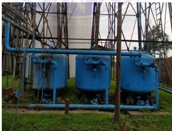
Gambar 3 61 Sand Filter
