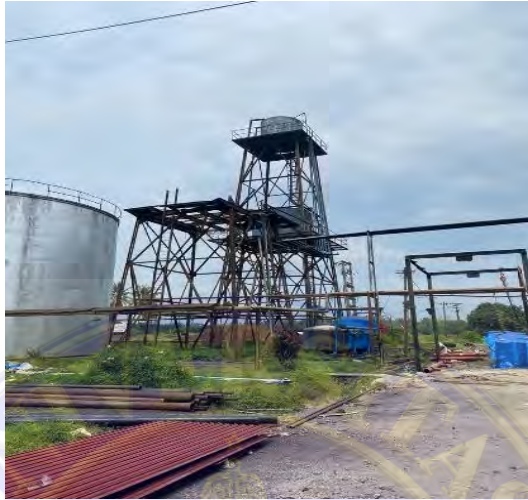
Gambar 3. 62 Water Tower Tank
