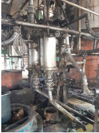
Gambar 3.14 Brush Strainer
