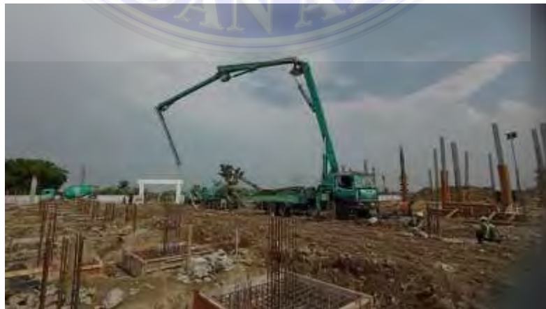
Gambar 3.3 Concrete Pump
