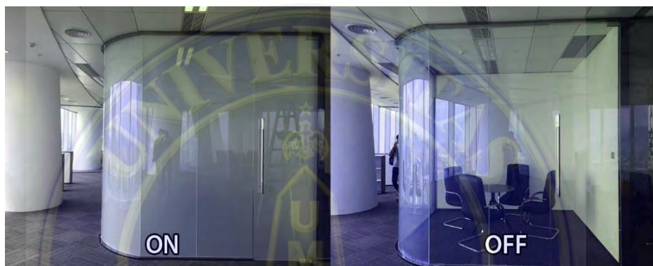
Figure 2. 1 Example of Electrochromic Glass Application
