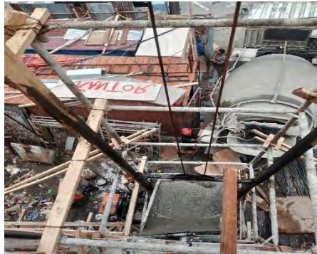
Gambar 3.15 Lift Beton
