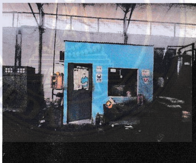
Gambar 3. 6. Ruang Kontrol Boiler
