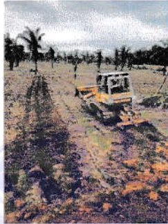
Gambar 4. Proses Ripping
