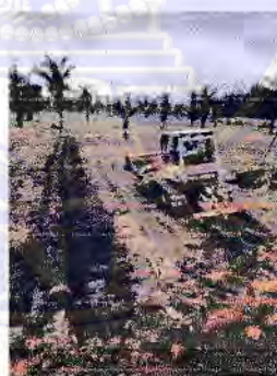
Gambar 4. Proses Ripping
