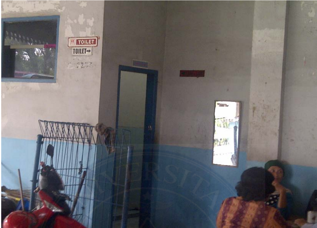
Gambar Kamar Mandi / Toilet
