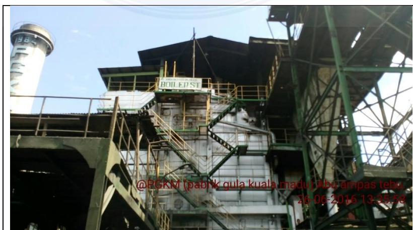
Tampak Mesin Boiler
