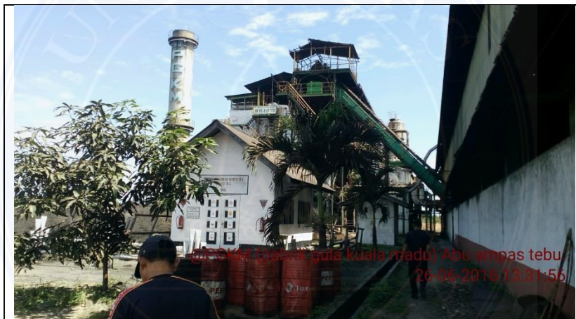
Tampak Mesin Boiler
