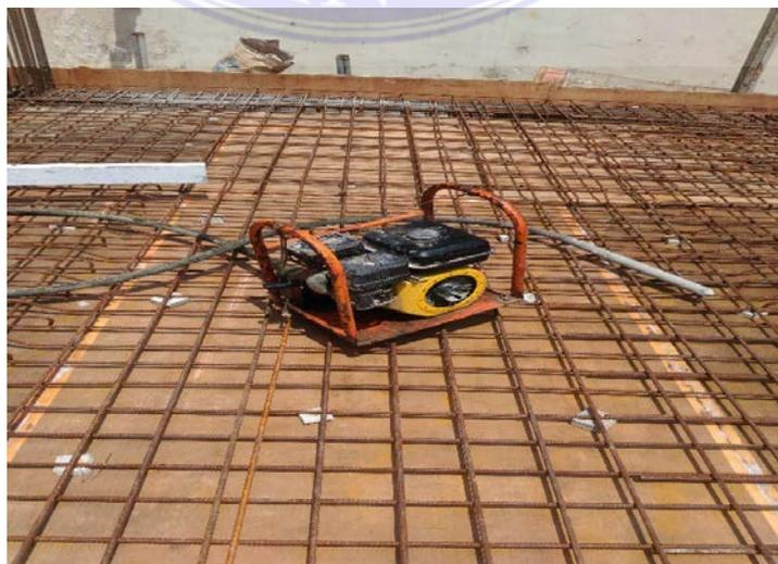
Gambar 2.1 : Concrete Vibrator
