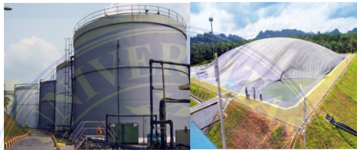
Gambar 2.2 Continuously Stirred Tank Reactor (kiri) dan Kolam tertutup (kanan). Sumber : Winrock Internasional 2015.
