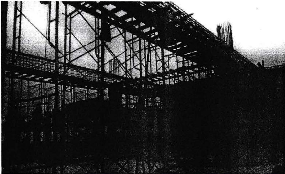
Gambar 3.18 Bekisting balok
