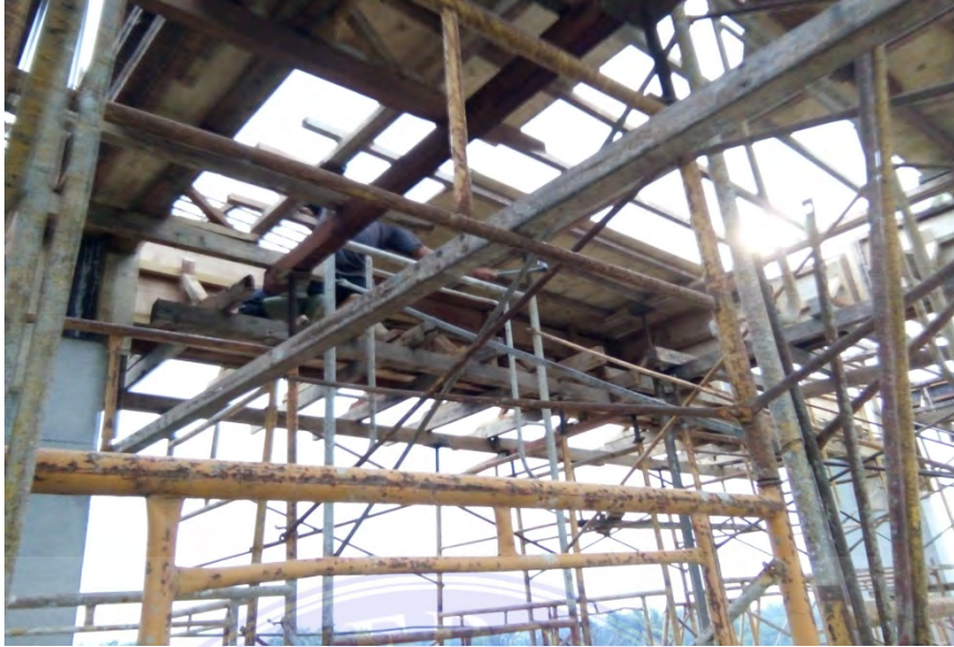
Gambar 3.2. Bekisting balok
