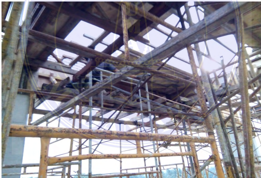
Gambar 3.2. Bekisting balok
