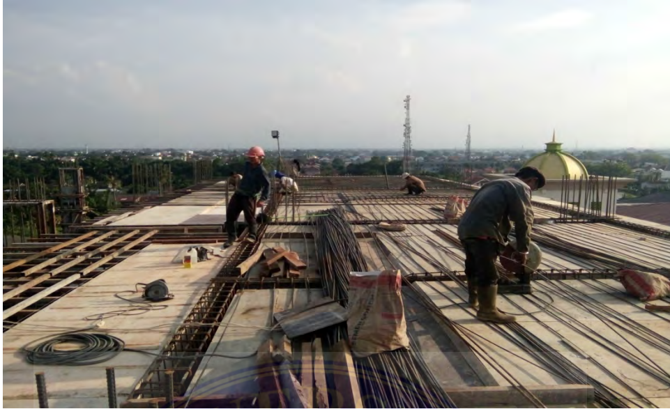
Gambar 3.3. Bekisting plat lantai
