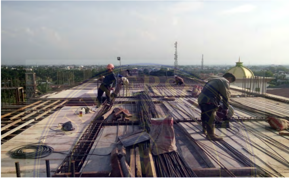
Gambar 3.3. Bekisting plat lantai
