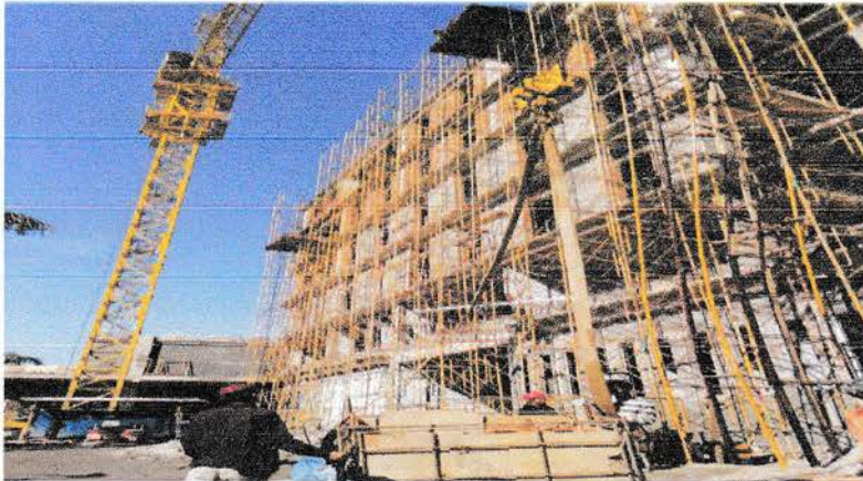
Gambar : Tower Crane
